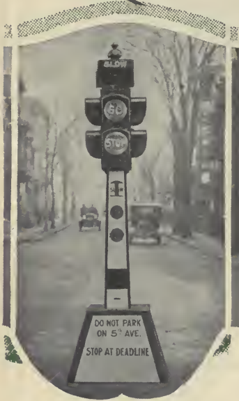
This signal placed in roadway at street intersection.
